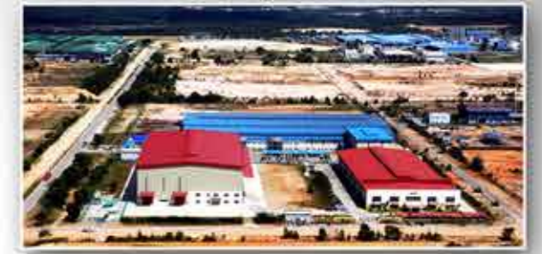
DYNAC SDN BHD main office / factory in Tanjung Langsat, Johor, Malaysia
